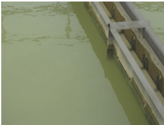
Figure 1. Poor settling (pH < 9.5)
